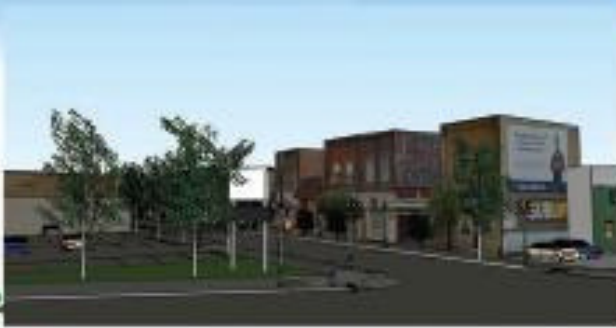
This Streetscape Project, located on Merchant Street between 4th and 8th Streets, has been designed to restore Ambridge's rich history while also addressing current and future needs. Much needed upgrades to the streetlighting, sidewalks, curbs, wheelchair accessible curb-cuts, and street trees will be performed as well as providing amenities such as benches, bicycle racks, and a park plaza. State-of-the-art lighting with low glare fixtures will provide improved visibility while highlighting seasonal displays and landscaping.
